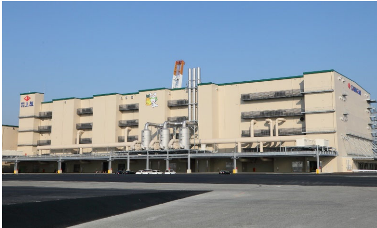
Fruit and vegetable distribution and processing center in operation in Kobe
